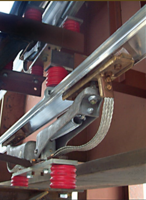
V Bar System with Corrugated Standoff Insulators
