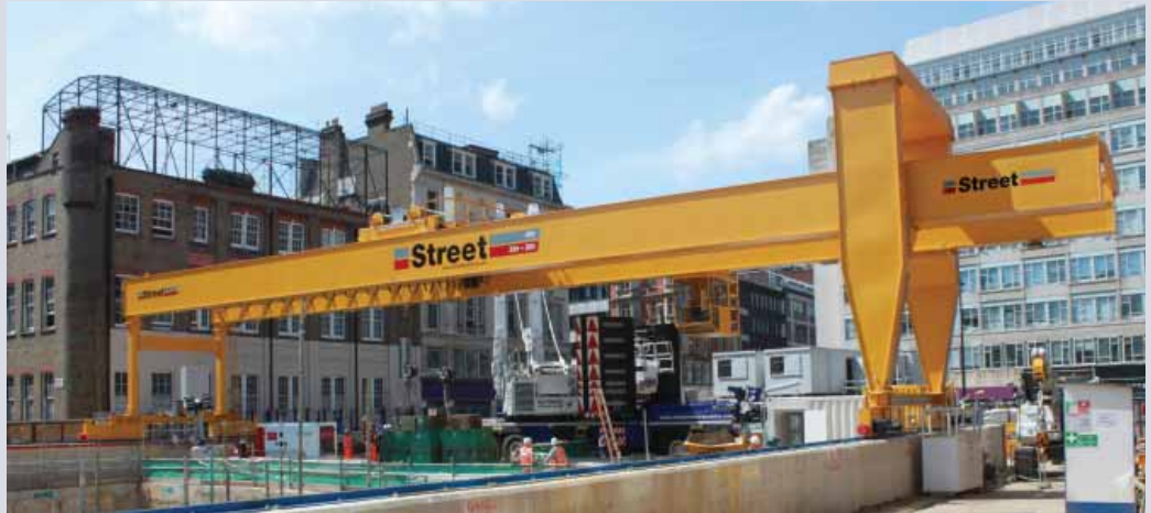
Spans in excess of 40m (130ft)
